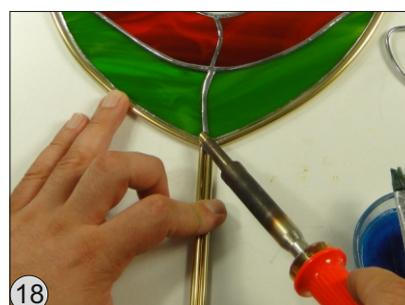
Set the first solder pad exactly, as shown to the joint.
