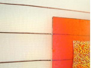
For a stronger construction please sold at both vertical sides two layers of reinforcing bar of 3,6x1mm ( 4220000 )
